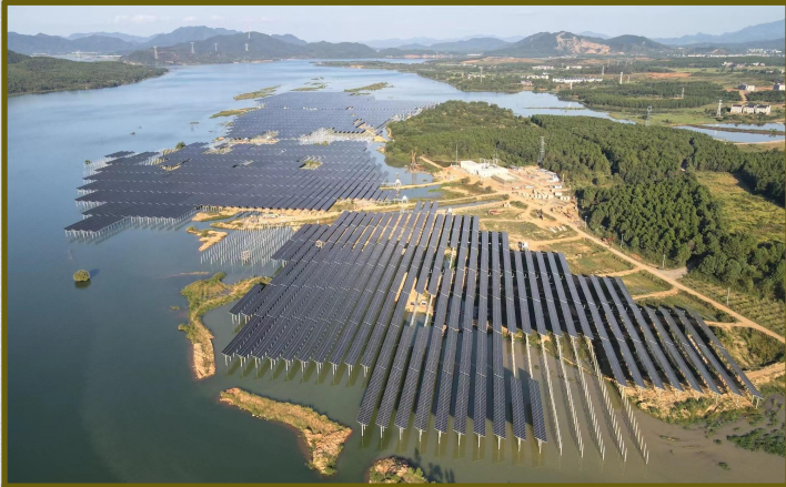
Jiangxi Water Power Station 55MWp
