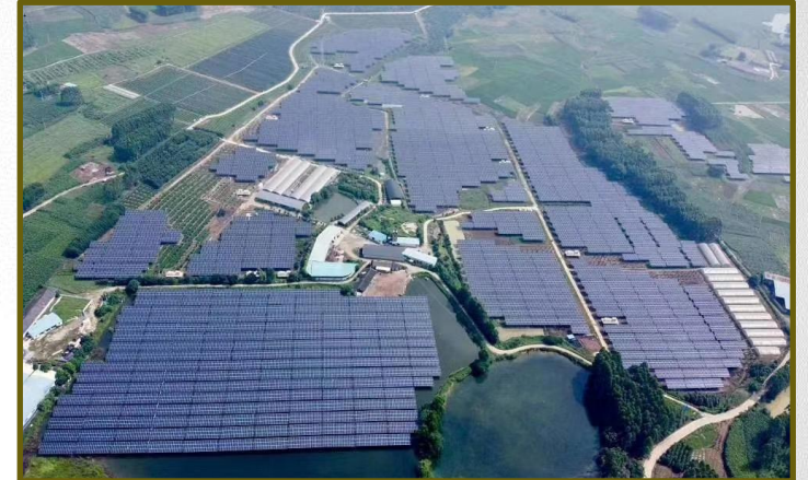
Zhejiang Floating Power Station 50MWp
