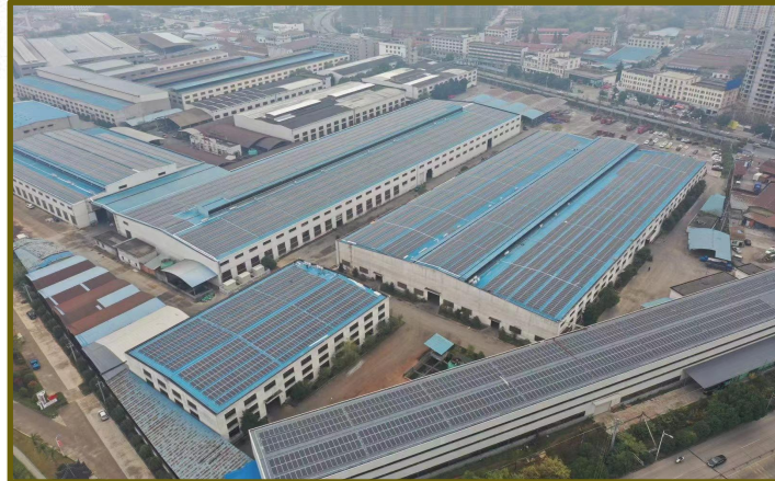
Suzhou Industrial and Commercial Power Station 10MWp
